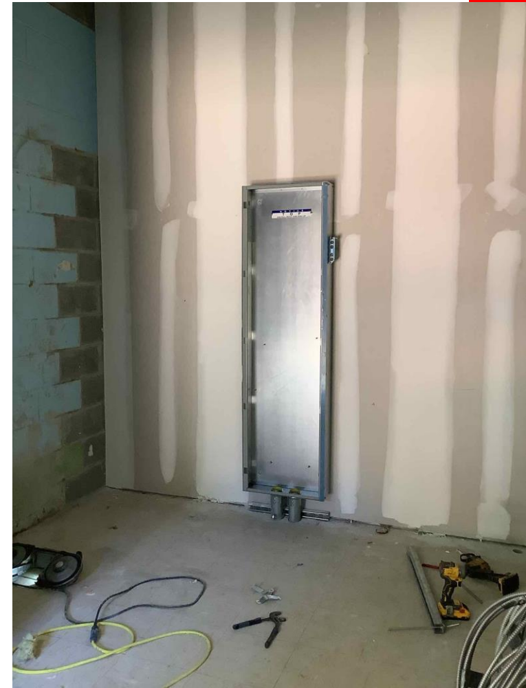
Panel board installation
